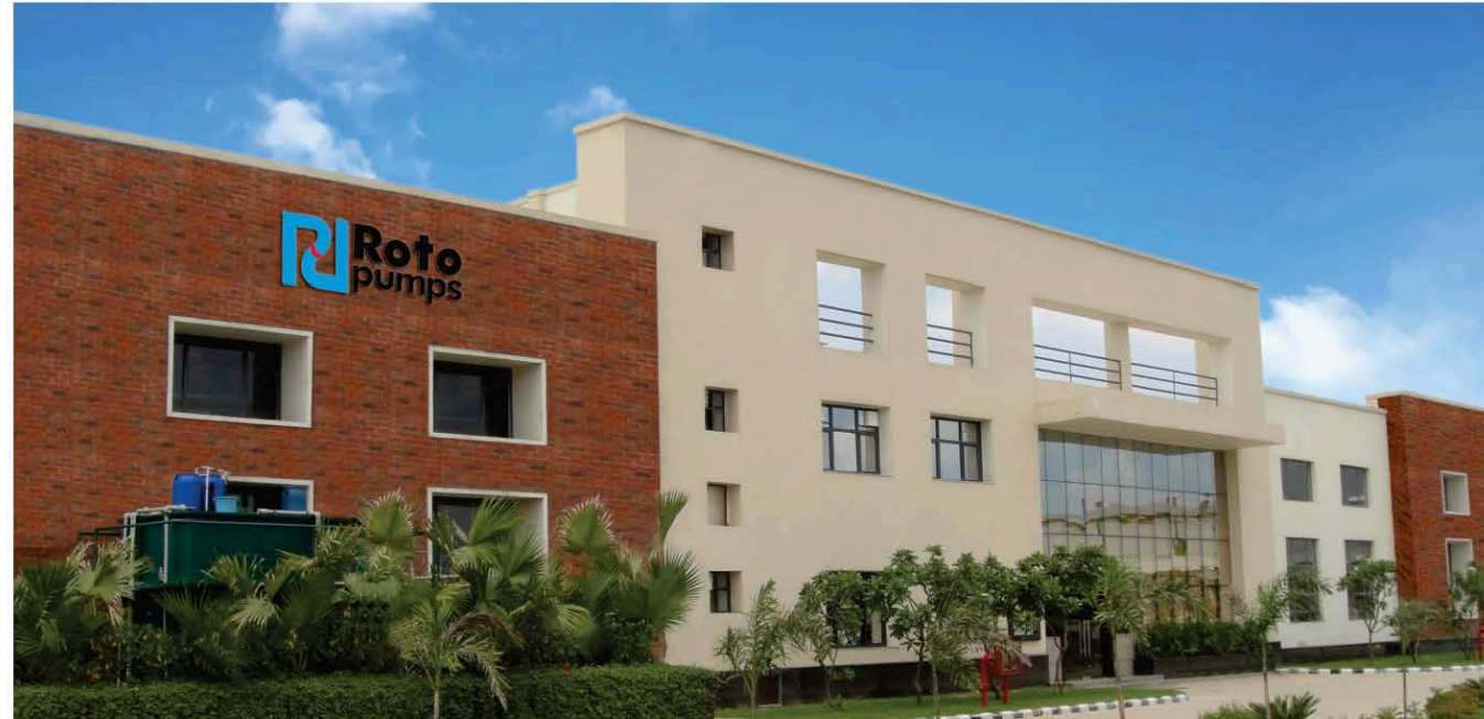
Roto Pumps Limited, Manufacturing Plant, India
