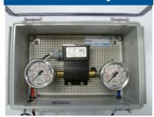
**OPTIONAL** Differential Pressure Switch Assembly for pressure differential backwashing.
